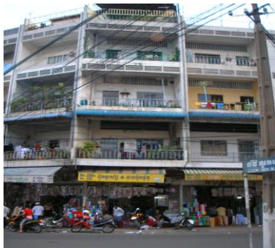
7. Shops at the first floor of a apartment
